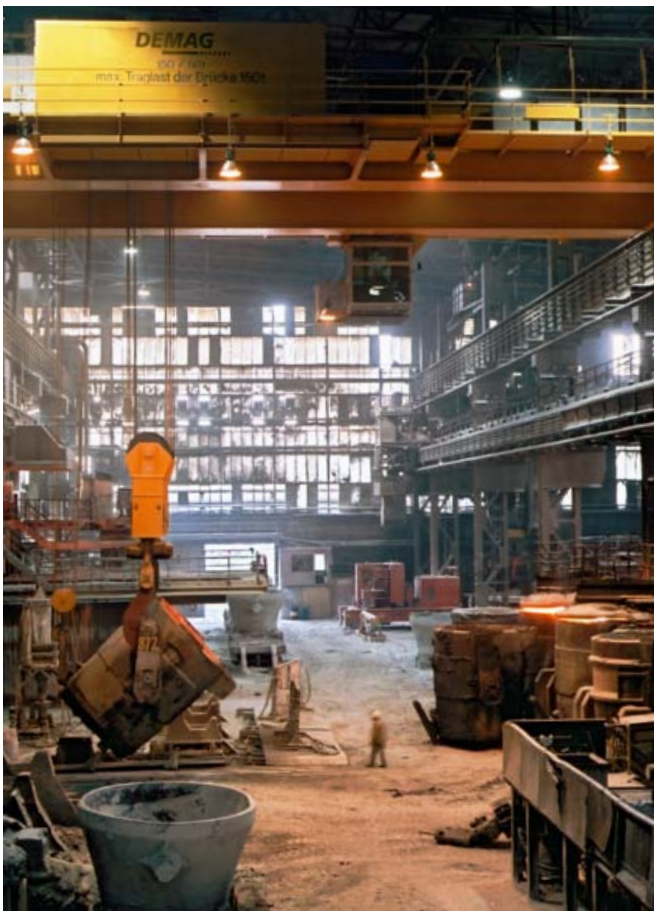
150/50-t two-girder overhead travelling crane for transport of molten materials in a German stainless steel factory
