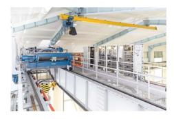
**41499-52:** Newly installed: the compact switchgear cabinets for the electric equipment were arranged on the walkway and a railing was installed for protection. Most of the components were raised to working level by the chain hoist installed on the I-beam girder.
